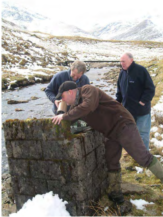
Figure 2: Old water level recorder installation on Cononish Burn
